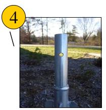
• 12" post should be slid into natural ground anchor first.
